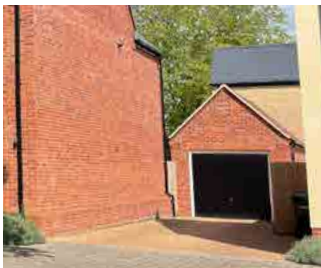
Driveway and garage.
