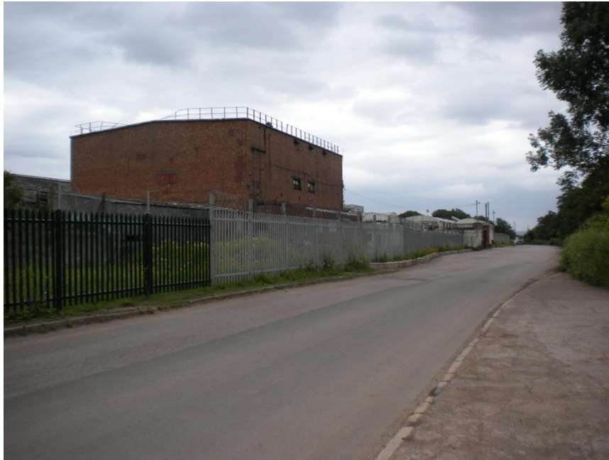
Photograph of Pine End Works looking south towards Harbour access road
