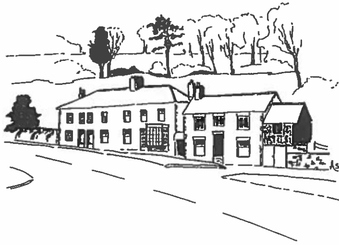
Fig 6 Viaduct Villas are a reminder of the industrial past and an attractive feature today.
