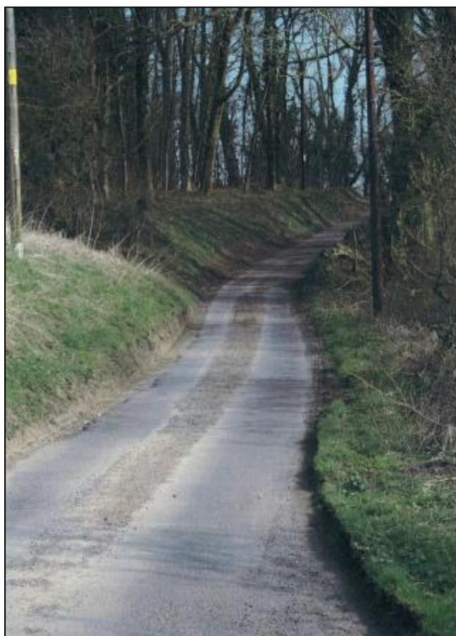
A typical fit for purpose rural unclassified road with some edge deterioration, over-riding, detritus and the occasional non-running lane pothole defect.
