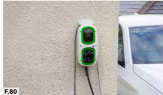
Figure 80: Electric charging points should be located discretely, where possible avoiding building façades visible from the road or public pathways to retain the character of the building.
